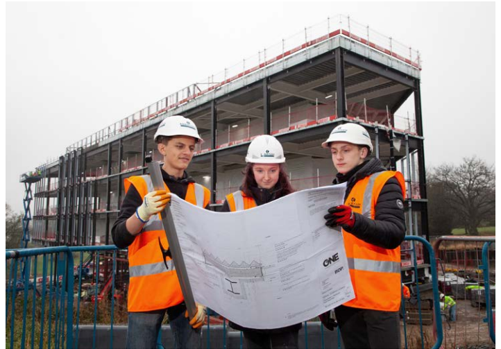
The BioHub build phase is supporting construction jobs in Aberdeen and encouraging new entrants to the industry, including construction apprentices from North East Scotland College (pictured from left) Mohamad Alhamdani, Jayden Dale and Owen Garner .
